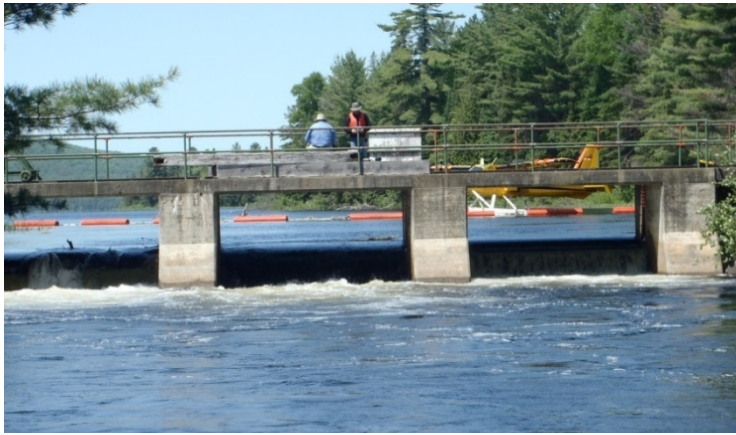
Figure 20. Booth Lake dam in 2013. This dam causes a 1 m water level difference between the lake and the downstream river so bars natural movement of large predator fish.
